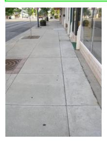
$\label{eq:Grade B-Minor Deficiency:} Grade \ B-Minor Deficiency:$  For instance, the sidewalk shown here has a cross slope greater than 2%.
