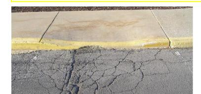
$\label{eq:GradeD-Multiple Major Deficiencies: The ramp shown here is too narrow, it is too steep, has a bad cross slope, and no detectable warning.$
