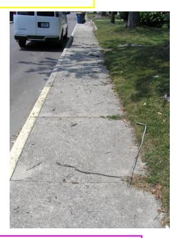
Grade D – Multiple Major Deficiencies: For instance, the sidewalks shown here are too narrow, they have joint displacements, rough/cracked surfaces, and gaps making it likely impassable by wheelchair, though a fit walker could still navigate the sidewalk.
