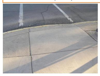
Grade C – Major Deficiency: The ramp shown here is too narrow, doesn't have a detectable warning, and has a joint displacement.
